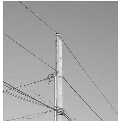
(b) Single-phase circuit, line-to-ground 7.2 kV.
